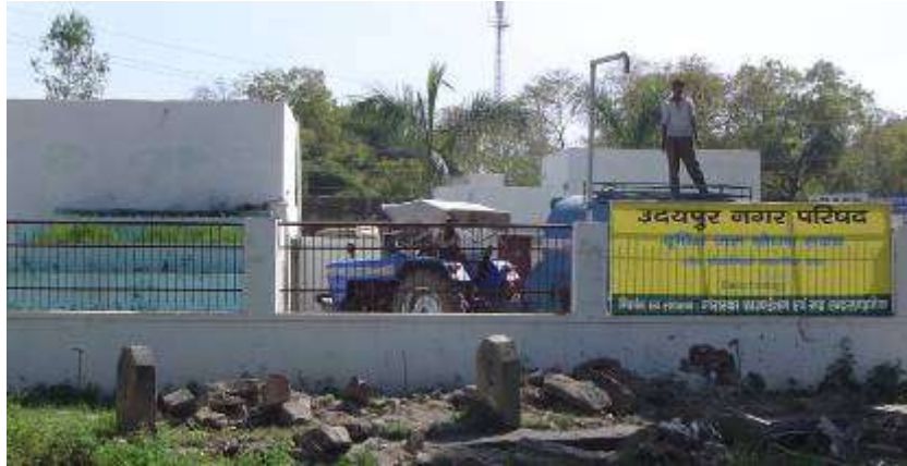
Installation of a 50,000 L/Day Waste Water Recycling Plant at Gulab Bag, Udaipur
