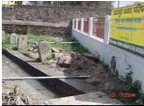
Grey water flowing through the drain
