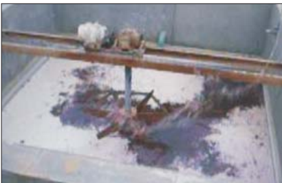
Spraying on ETP plant
